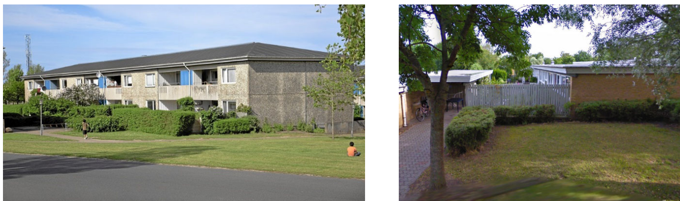
Figure 3. Apartment block ( left ) and detached house ( right ) before renovation.
