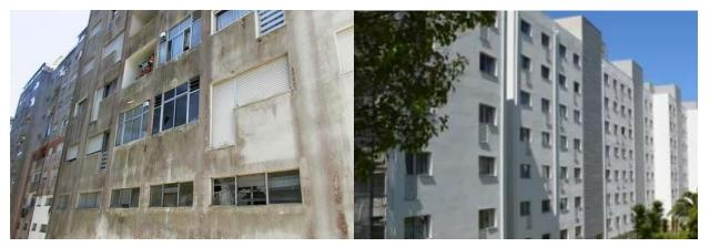
**Figure 32.** Façade in Vila D'Este district before renovation (left) and after renovation (right). Source: Gaiurb, from: http://www.cm-gaia.pt/fotos/editor2/a-nova-vila-deste.pdf
