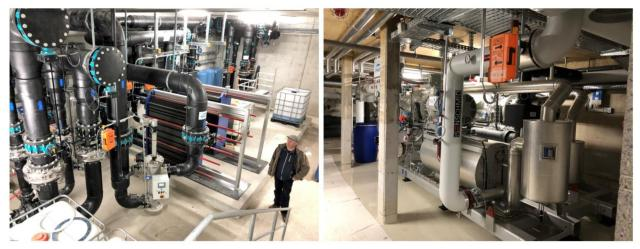
Figure 52. Right: Lake-water pumping station. Left: 1 MW Heat pump. Source: Corporation Weggis.
