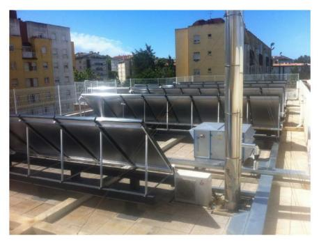
Figure 36. Solar thermal system installed in the pool roof. Source: Lisboa E-Nova.
