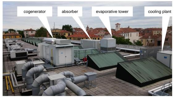
Figure 23. External view of the roof with actual localization of the trigeneration plant on the roof of the Ex Cotonificio. Source: University IUAV of Venice.
