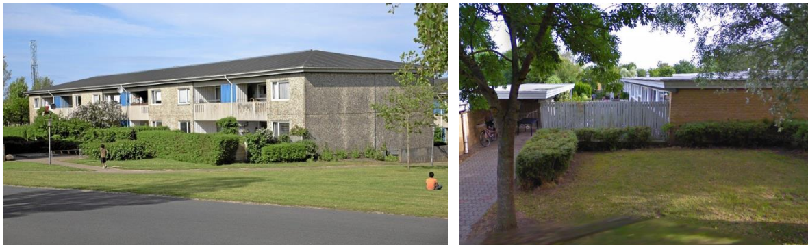
Figure 2. Apartment block (left) and detached house (right) before renovation.
