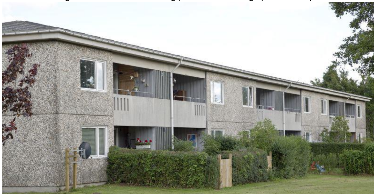
Figure 6. Typical prefabricated concrete building.
